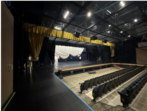
CHS – Auditorium Stage Flooring
