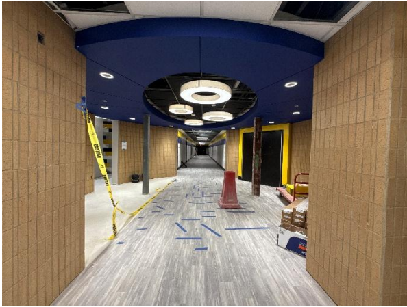
CHS – Auditorium Lobby Flooring In Progress
