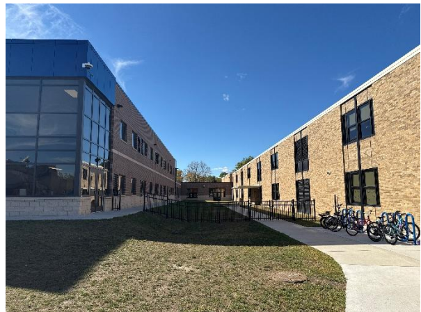
Campus – New Dog Fence Gate between CMS & CES
