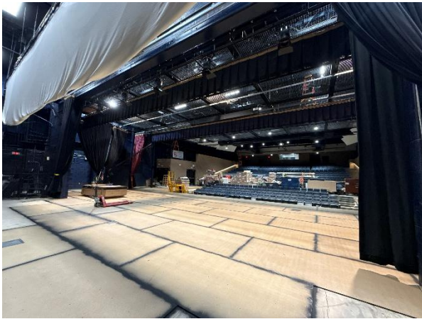
CHS – Auditorium Stage Flooring In Progress
