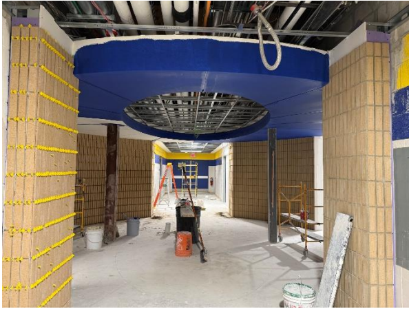
CHS – Auditorium Lobby Thin Brick In Progress
