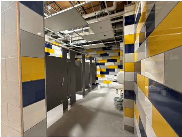
CHS – Auditorium Lobby Toilet Room Plumbing Fixtures In Progress
