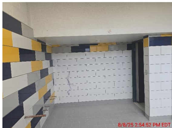
CHS – Bathroom Tile & Grout Install In Progress
