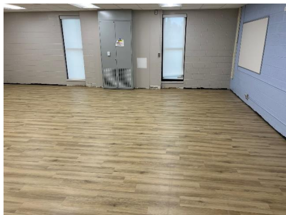
CHS – Classroom LVT Flooring Install In Progress
