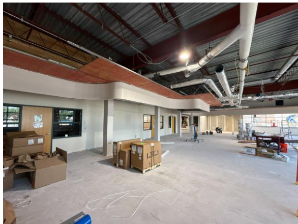
CHS – Media Center Baffle System In Progress
