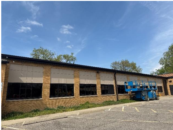
ECC – Exterior Metal Composite Panels In Progress
