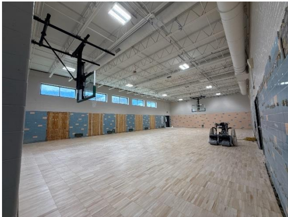
ECC – Gym Flooring In Progress
