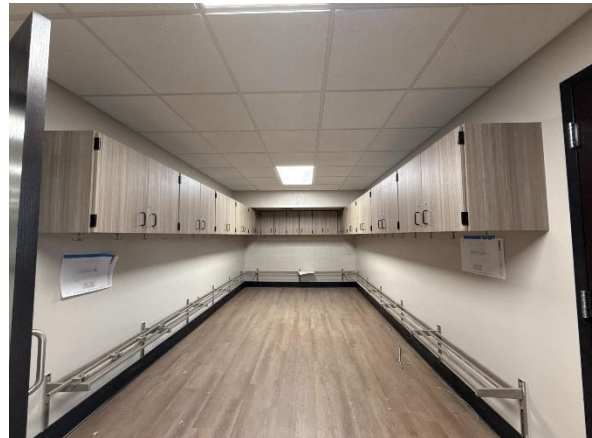
ECC – Closet Coat & Boot Racks In Progress
