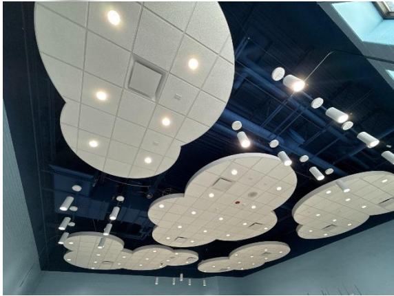
ECC – Ceiling Clouds In Progress
