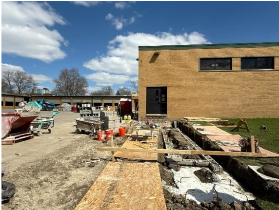
ECC – Site Work In Progress
