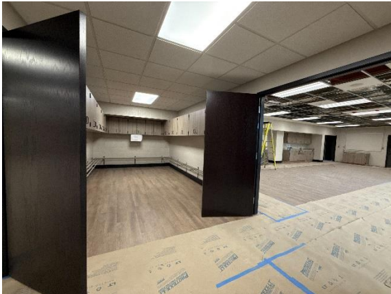
ECC – Closet Casework & Doors In Progress
