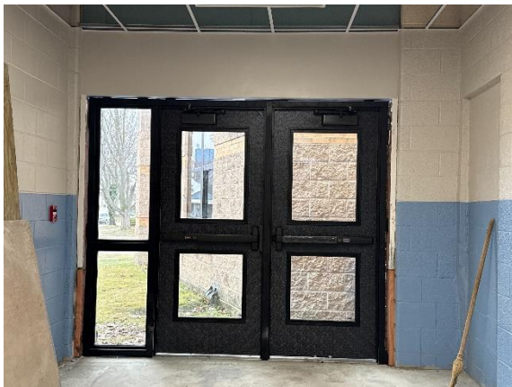
ECC – Exterior Corridor Doors In Progress
