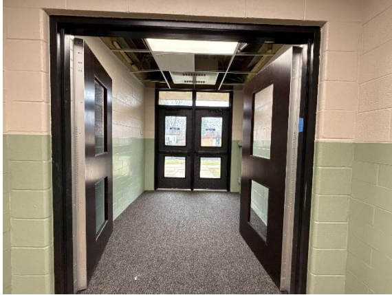
ECC – Corridor Carpet Flooring In Progress
