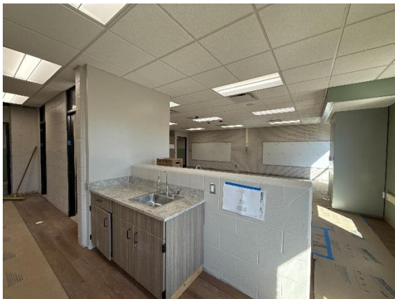
ECC – Classroom Sink Fixtures & Markerboards In Progress
