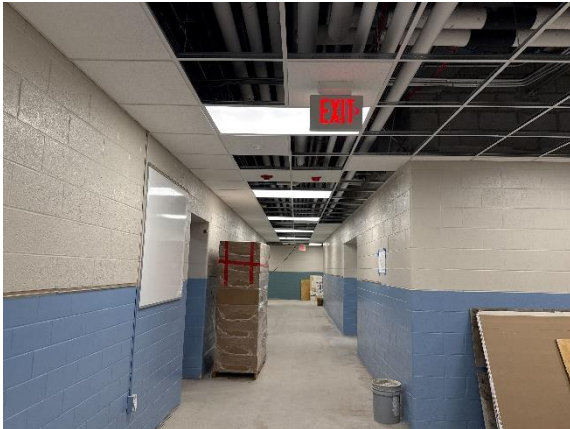
ECC – Egress (Exit Signs) In Progress
