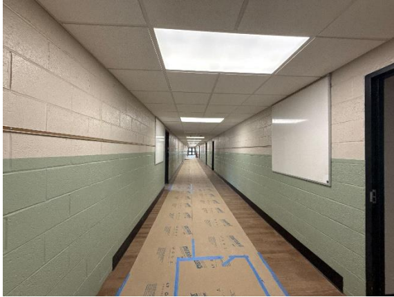
ECC – Corridor Floor, Base, & Markerboards In Progress
