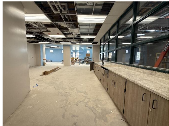
ECC – Media Center Casework In Progress
