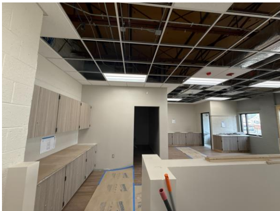
ECC – Casework & Flooring Install In Progress
