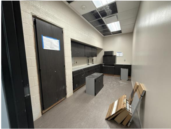
ECC – Main Office Printer Space In Progress
