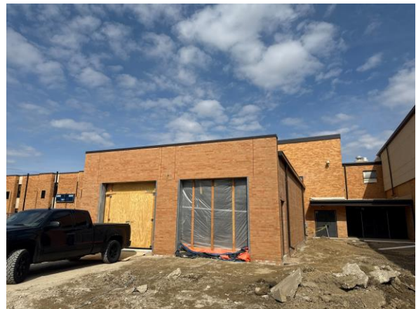
CHS – Maintenance Garage In Progress
