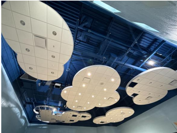
ECC – Cafeteria Clouds Lighting In Progress
