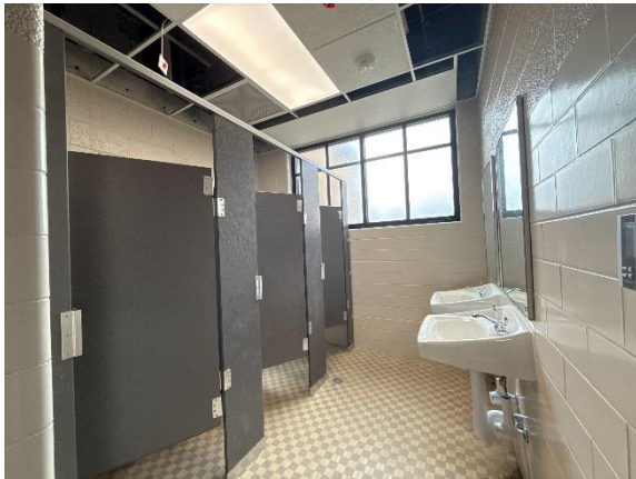
ECC – Toilet Partitions Install In Progress
