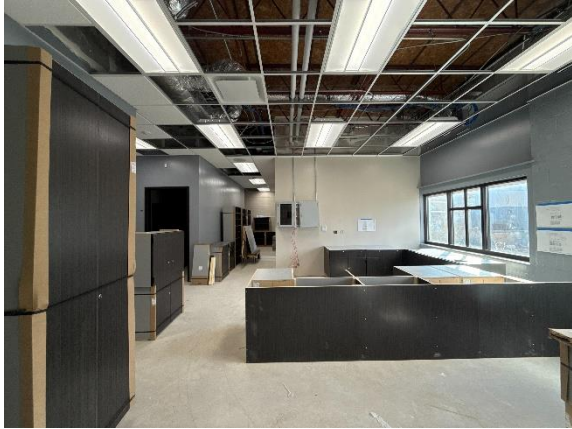
ECC – Casework Install In Progress
