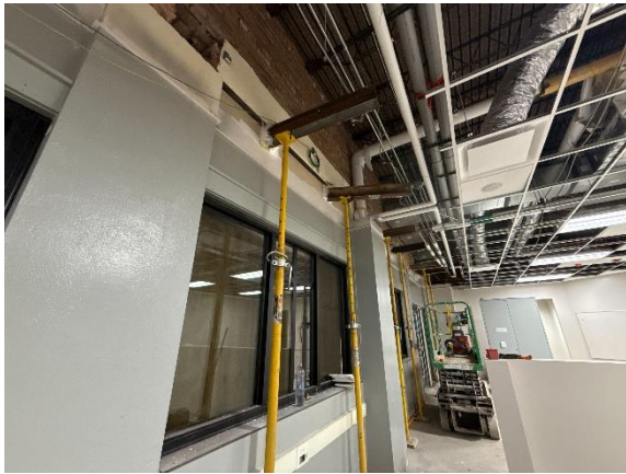
ECC – Lintel Repair In Progress
