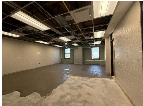
ECC – Floor Prep In Progress
