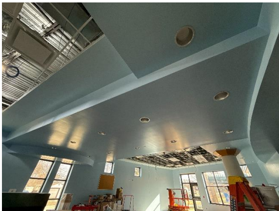
ECC – Media Center Lighting In Progress
