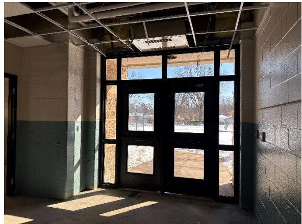
ECC – New Exterior Doors Install In Progress
