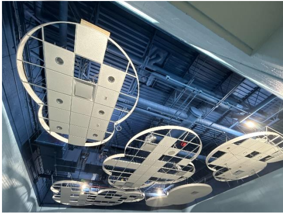
ECC – Cafeteria Clouds Lighting In Progress
