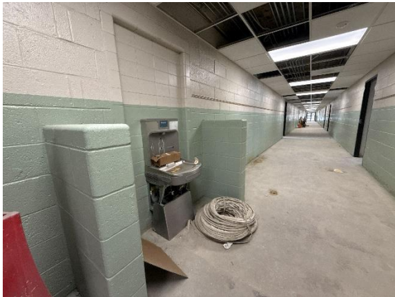
ECC – Water Fountain Install In Progress
