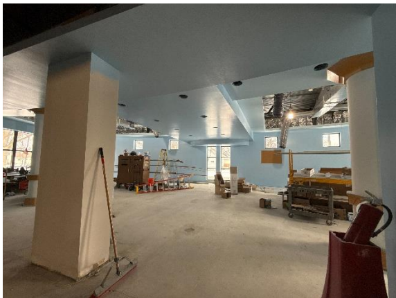
ECC – Media Center Painting In Progress
