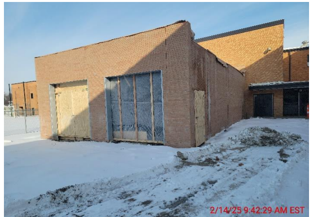
CHS – New HS Maintenance Garage In Progress
