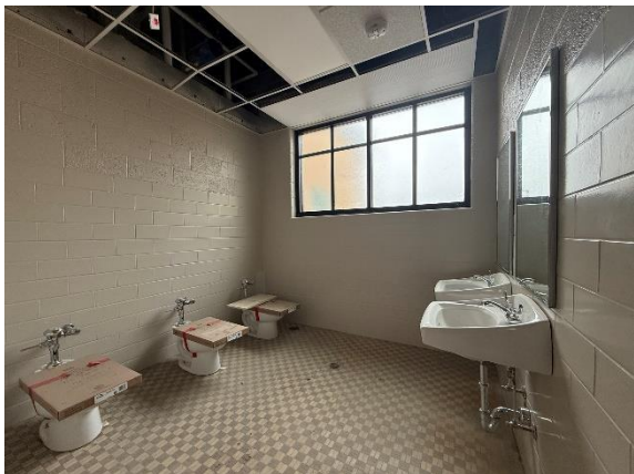
ECC – Installing Toilet Fixtures In Progress
