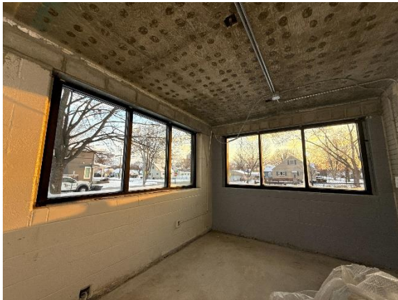
ECC – South Side Lintels In Progress
