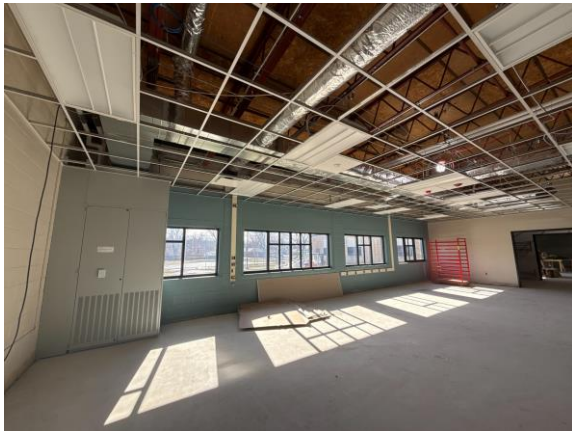
ECC – South Side Classrooms In Progress
