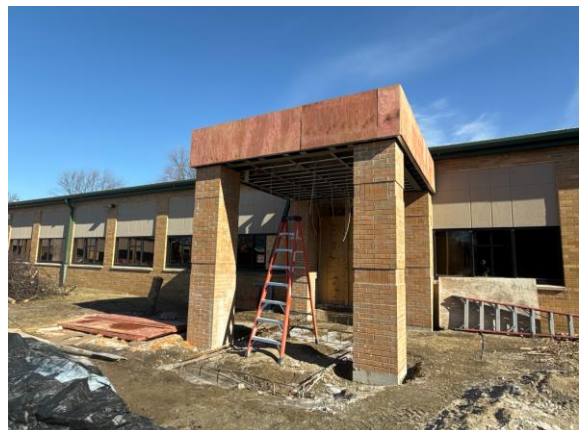
ECC – Main Office Exterior Entrance In Progress
