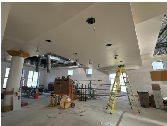
ECC – Media Center Interior Lighting In Progress
