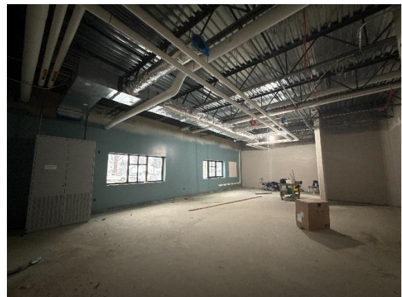
ECC – Painting In Rooms & Corridors In Progress
