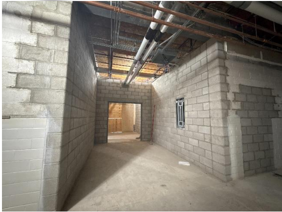
ECC – Main Entrance Corridor In Progress
