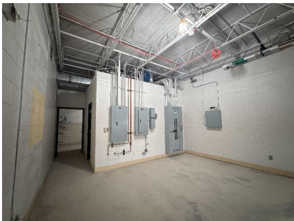
ECC – Electrical Receiving Room In Progress
