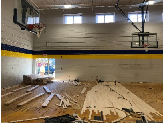
CES – Gym Addition Wood Floors Install In Progress
