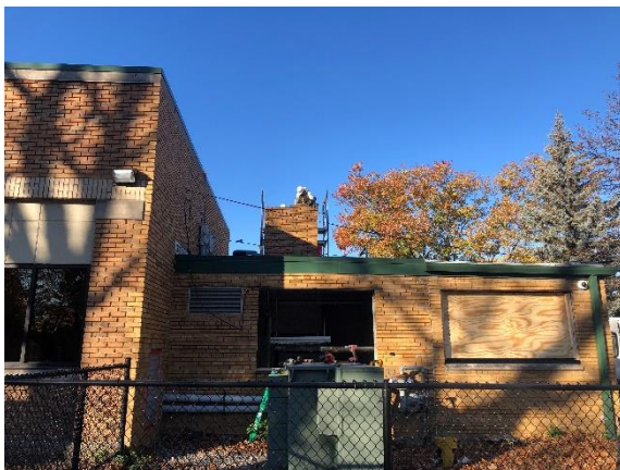
ECC – Chimney Demo & Window Install In Progress
